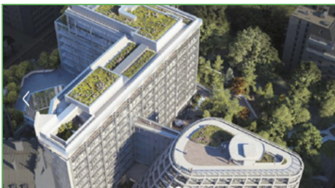
Aerial View of the BIOME Building
